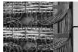
Combination Organizers systematically deliver cables horizontally to 110 clips for termination. Vertical Organizers form a rear channel for cables while Vertical Control Brackets help contain them.
